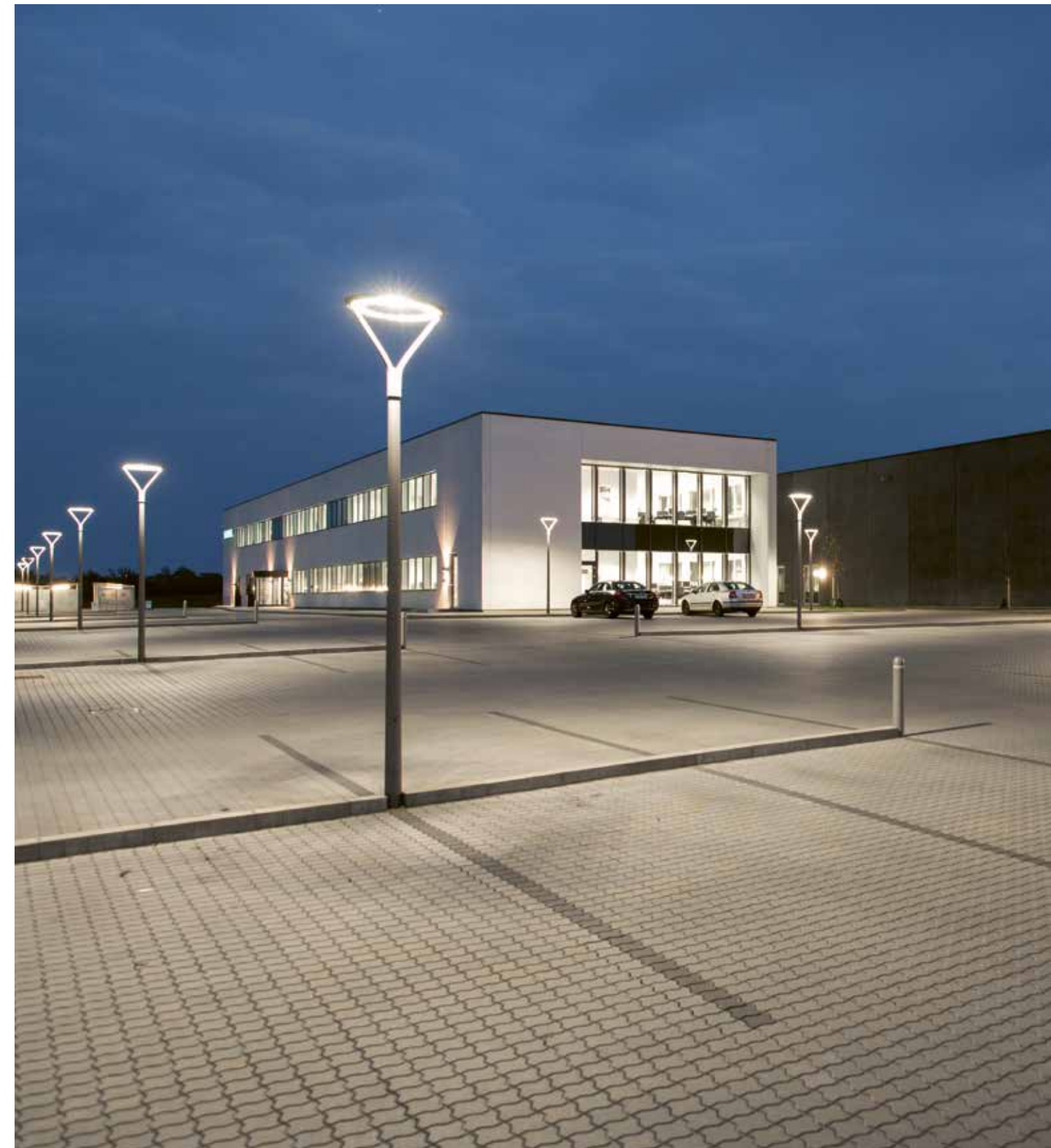
Project: Siemens Flow Goods, Sonderborg, Denmark Product: DL ® 20
