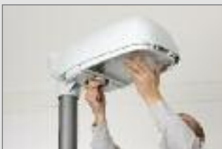
1. Open the luminaire: a twist-lock catch locks the luminaire cover.
