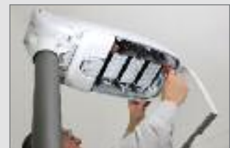
3. Loosen the connection screws of the gear tray.
