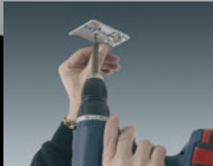
Fastening of quick mounting plate with one screw
