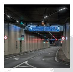
Kaisermühlentunnel, Vienna/Austria, 2018 Interior zone lighting with linear compact luminaires
