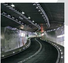
Tunnel, Lungern/Switzerland, 2012 Entrance zone and interior zone lighting with symmetric compact luminaires, the first LED tunnel in Switzerland
