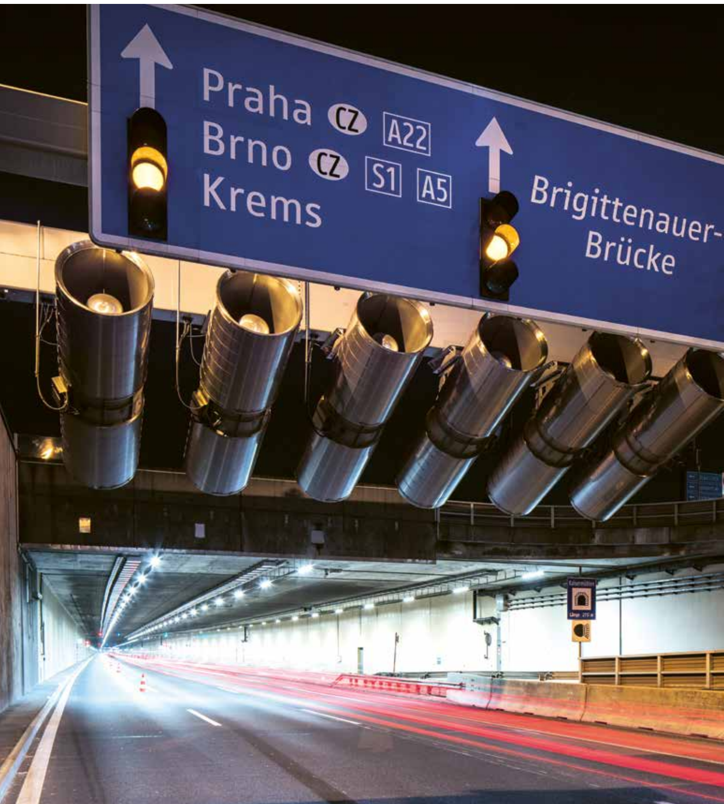
Project: Kaisermühlentunnel Vienna, Austria Product: Tunnellight TL 23
